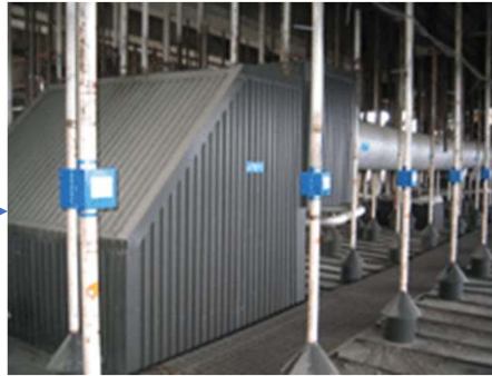
Direct deposit accumulation measurement with StrainGauge (SG)
